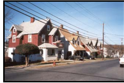
These Single-Family Residences along Oak Street on the edge of the Downtown Walden Business District provide a distinct and well-defined edge to Downtown Walden. Photo by AJS
