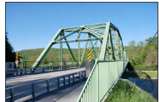
Above (top to bottom): Gateway to the Village of Hancock and New York State upon crossing the bridge over the West Branch of the Delaware River; unsightly Village-owned property with dilapidated building that lies to the right of the “Welcome to New York Sign”; view of bridge looking toward Pennsylvania. The Bridge provides an aesthetically entrance into the Village. The Village-owned property should be redeveloped as a waterfront park.
