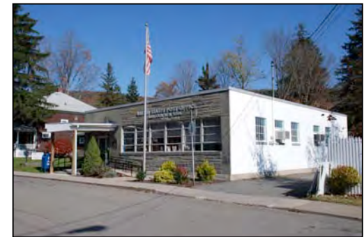
Above (top to bottom): The Louise Adelia Read Memorial Library on Read Street; the 1909 Opera House [aka Old Capital Theater] on East Front Street; and Post Office on Wheeler Street are important civic institutions within Downtown. Having these civic institutions Downtown enhances the vitality of the business district.
