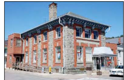
Above (top to bottom): U.S. Post Office on Wheeler Street; Lourdes Primary Care Clinic on East Front Street; and NBT Bank on West Main Street. Each of these entities provides important services that are used by the general public on a daily basis. They draw customers to the Downtown Business District on a regular basis that in turn helps to support local business that benefit from the additional pedestrian traffic.
