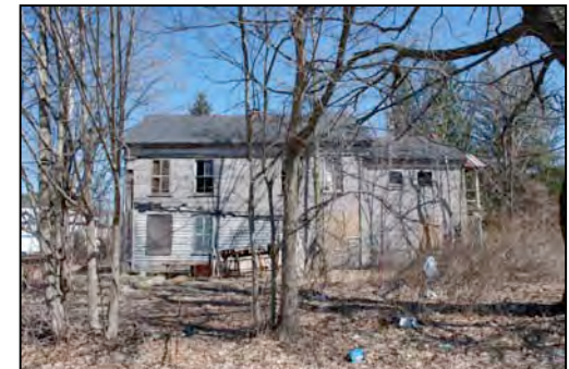
Above (top to bottom): Beautifully restored Queen-Anne house on Leonard Street that is one of a number of large single-family homes that are being restored in the Village; small Cape on Upper Pennsylvania Avenue with some minor deficiencies; and dilapidated house on Wheeler Street (south of railroad tracks) that is a blight on surrounding properties and should be removed.
