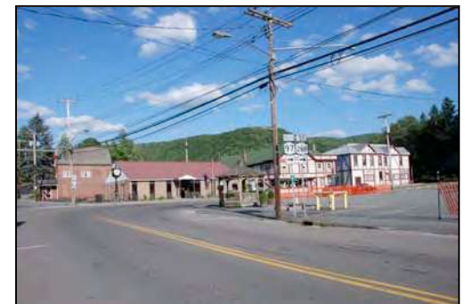
Above (top to bottom): Former Great American Supermarket Building that has become a blight on the Downtown Business District; view of Great American site looking from East Front Street to West Main Street; and view of Great American Site looking from West Main Street toward Read Street. This site, or a portion thereof, would make the ideal location for a Village Square.
