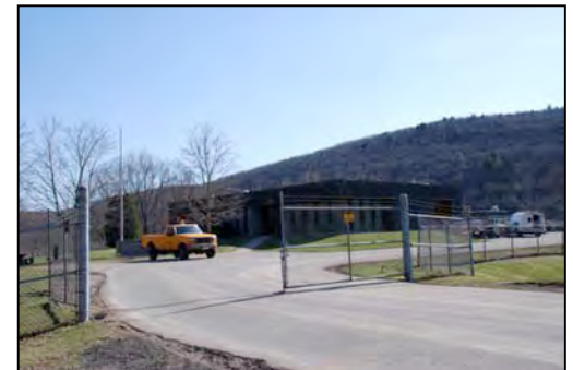
Above (top to bottom): Village reservoir at the end of the Golf Course Road Extension; another view of reservoir; and view of Village-owned Waste Water Treatment Plant at the end a LaBarre Street south of the Village. The Village has excess capacity to accommodate new growth the water and sewer lines already serve the area where growth is likely to occur.
