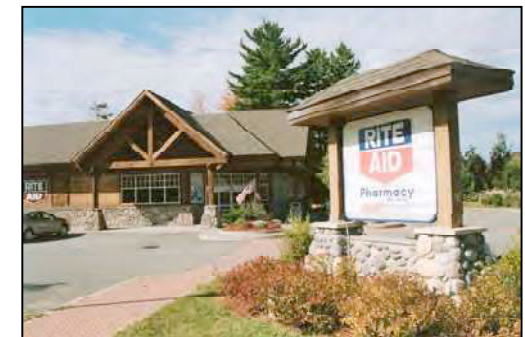
Above (top to bottom): Rite Aid Pharmacy in Camden, ME as an example of chain store that respects character of this historic community; existing Rite Aid Pharmacy in Hancock; and Rite Aid Pharmacy in Lake Placid, NY. There is little that can be done to address how the existing Rite Aid is situated, however, a façade renovation and new signage that incorporated elements of the Lake Placid Store would be more in keeping with character of Hancock, NY.
