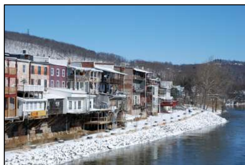
Above: View of Property looking southeast toward the site; view from Front Street looking across site to the Susquehanna River; view of Owego Riverwalk looking east from just behind the subject site and view of site from NYS Route 96 Bridge.
