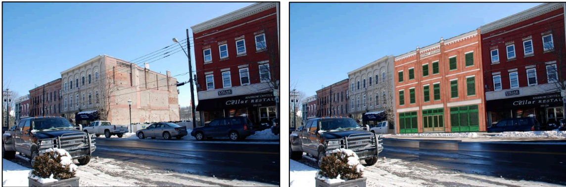
Above (left to right): Photo taken in February of 2011 showing the Property (i.e. 202-204 Front Street), which is presently a vacant lot followed by a photo simulation of the Gateway Building erected on this site. The construction of the Gateway Building will help to re-establish the cohesive building fabric of the River Row along Front Street, while restoring business and residential opportunities on the Property.
