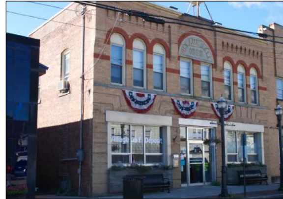
Do This: Village Hall circa 1899 has retained many of its original architectural elements. Although windows were replaced, the style and openings were maintained. The Base-Middle-Top of the Village Hall facade is distinguished by the door and window openings at the base and facade articulation and openings along the second floor.
