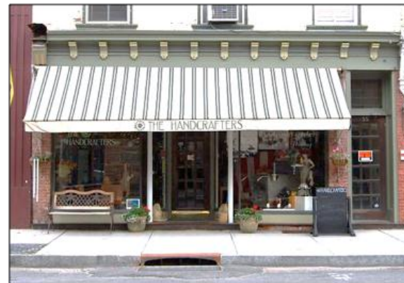
Do This: The Handcrafters. The recessed entrance to the storefront is well defined and the owners have used awnings to help accent the entrance. The entrance to second floor is located in front right side of building façade, but is separate and distinct from the commercial business entrance. A lower cornice helps to distinguish the first floor from the upper floors. There is also a high percentage of door and window openings on the first floor.
