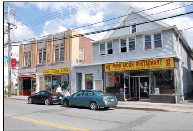
Above: The Ming Liquors & Wines building has a flat roof with a decorative upper cornice that complements adjacent buildings; the Ming Moon Restaurant has a hip roof. It appears that the upper stairs front porch was enclosed -concealing the original design.
