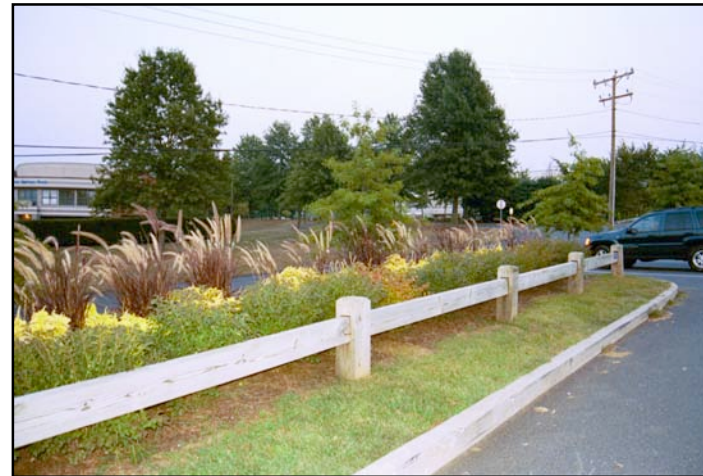
Above: CVS-Southbury, CT. The wood guide rail and abundant landscaping soften the edge of this parking lot.
