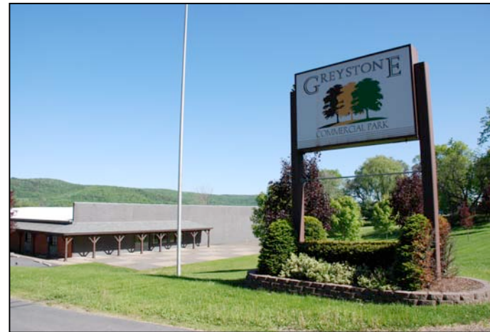
Above: Greystone Commerce Park - Hartwick, NY. Building setback, landscaping and projections help to soften this industrial building.
