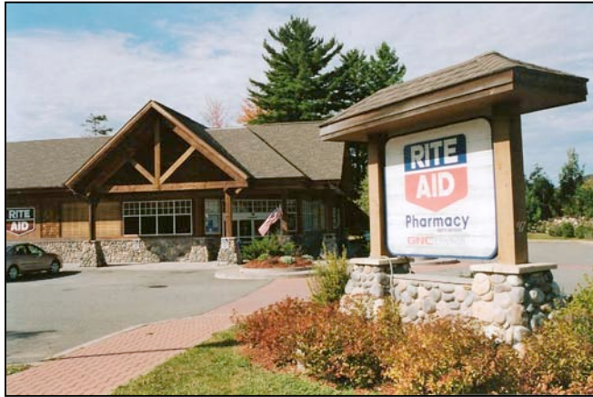
Above: Rite-Aid Lake Placid - Appropriate Design. This Rite-Aid incorporates a sloping roofline, projections, landscaping and the use of stone and heavy timber material. Such elements are encouraged in Fallsburg.
