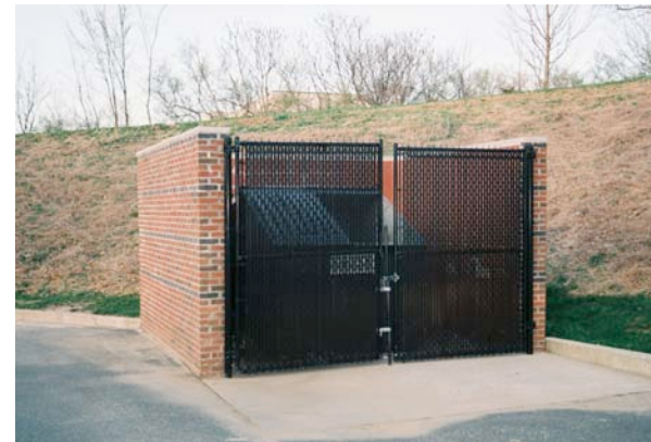
Above: Appropriate means of enclosing a trash container.
