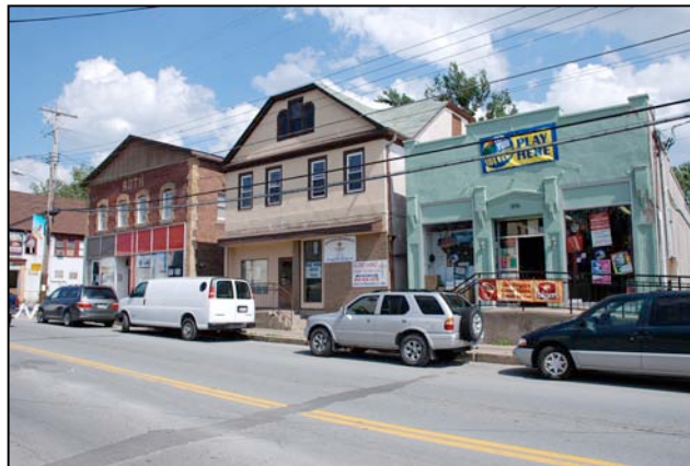
Above: There is an eclectic mix of rooflines in South Fallsburg including gable, hip and horizontal. The building to the left was originally built with a flat roof - the gable roof later added; middle building showing hip roof and building far right with a flat roof concealed behind a parapet wall.
