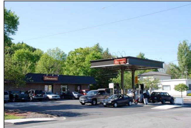
Above: Stewart's Shop in Cooperstown, NY. The muted colors of the gas canopy coupled with subtle signage with gooseneck lamps allow this retailer to complement the historic character of the community.
