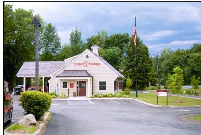
Above: Ulster Savings Bank on Route 209 in Marbletown, NY. The sloping roofline, large setback from Route 209, generous landscaping and placement of parking to the rear of the site helps to protect the viewshed from Route 209.
