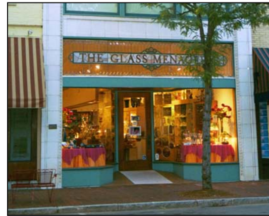
Above: The Glass Menagerie in Corning, NY incorporates the classic elements of a traditional storefront on Main Street. Note the well-defined bulkhead, display window and transom as well as the recessed entry.
