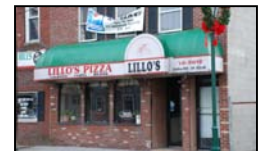
Above: An example of a "Fixed quarter-round awning sign" that is inappropriate to building design.
