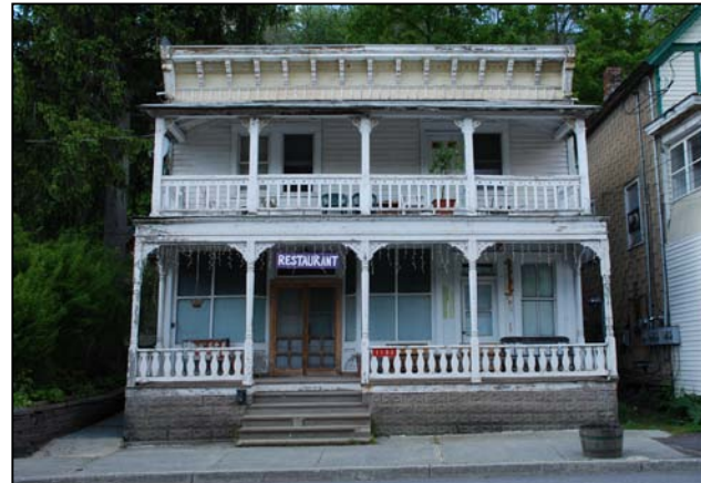
Above: Restaurant at 1103 Main Street with a flat roof. Original architectural features include a decorative upper cornice, front porches with original baluster & balustrade and large display windows on storefront. The renovation should be limited to repainting and repair of any exterior elements in disrepair.
