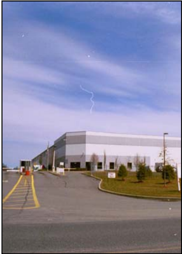
Above: Inappropriate entrance with no projection or recess to define the building entrance.
