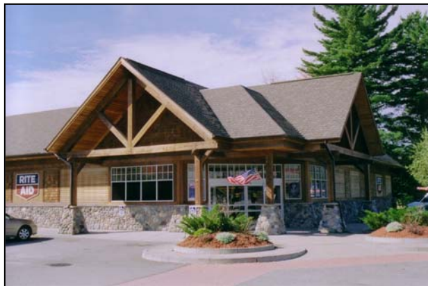
Above: Rite Aid-Lake Placid, New York. An example of well-defined building entrance that is designed to the human scale.
