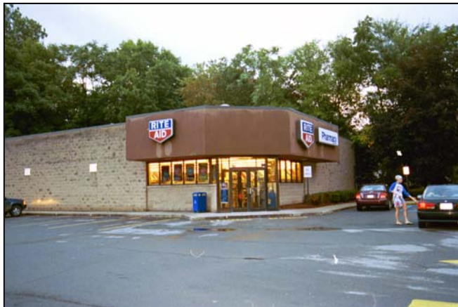
Above: Rite-Aid Ellenville - Inappropriate Design. Standard box-like buildings shall be prohibited in the Town of Mamakating.
