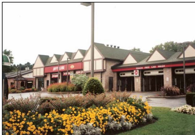
Above: Jiffy Lube/Hoffman Car Wash in the Town of Colonie, NY. The building incorporates dormers, changes in roof form, and changes in colors and materials to break up the mass of the building. Generous landscaping and subdued signage also enhance the appearance of this retail establishment.
