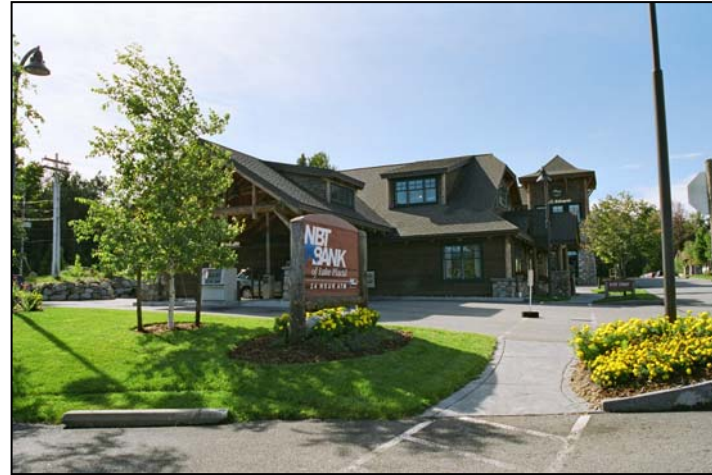
Above: NBT Bank-Lake Placid, NY. Variations in the roof line, recessed entry, and use of stone and timbers make this building visually appealing.
