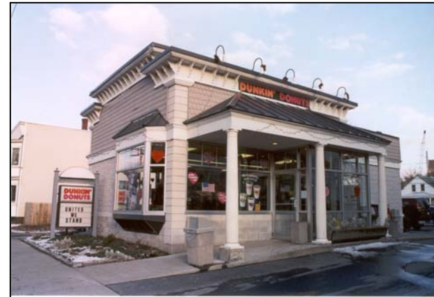
Above: Dunkin' Donuts- Rensselaer, New York. Example of well-defined building entrance that is designed to the human scale. This building incorporates a portico to help to define the human scale of the entrance.
