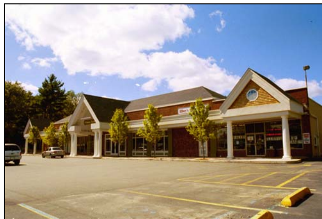
Above: Eagle Plaza in Monticello, NY. This is an example of a new façade that incorporates dormers, recesses and projection to break up the mass of the building. Good example of adaptive reuse of older retail center.
