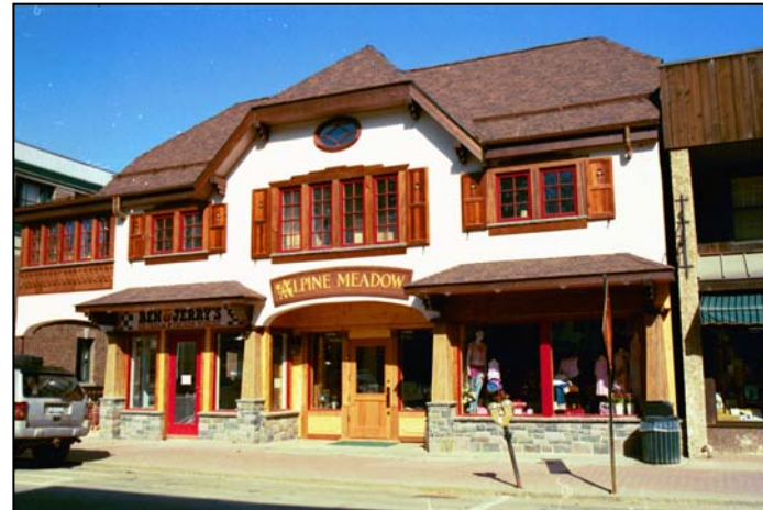
Above: Ben&Jerry's-Lake Placid, NY. Variations in the roof line, recessed entry, and use of stone and timbers make this building visually appealing.
