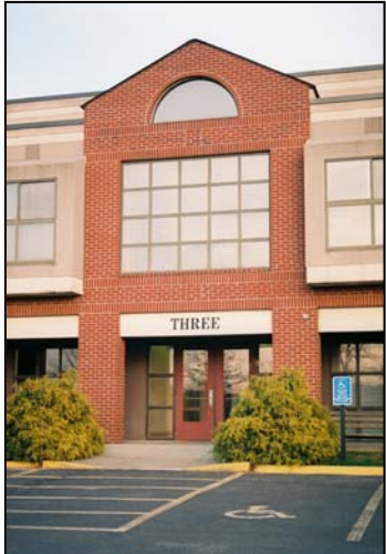
Above: Appropriate entrance that incorporates projections and a recess to define the building entrance.
