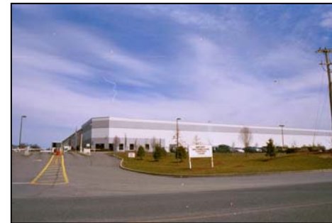
Above: Inappropriate entrance with no projection or recess to define the entry.
