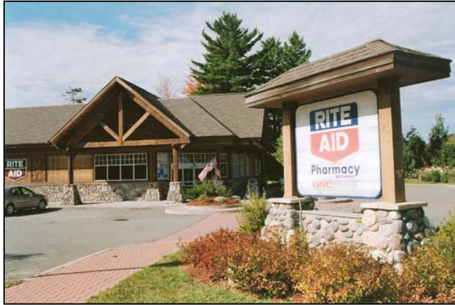
Above: Rite-Aid Lake Placid - Appropriate Design. This Rite-Aid incorporates a sloping roof line, projections, landscaping and the use of stone and heavy timber material. Such elements are encouraged in Mamakating.
