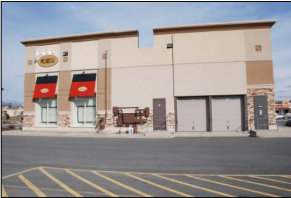
Do This: In this example, the trash containers for the AT&T and Talbots Building is fully enclosed within the building itself. The entrance to the refuse collection area is behind the garage doors, with access to the service lane. However, more thought should have been given to the utility boxes, which have a “tacked on” look.
