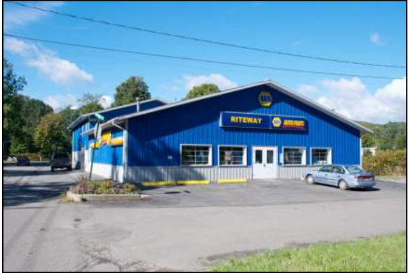
Don’t Do This: The Riteway Napa Auto Parts store in the Village of Deposit, NY represents the wrong way to design a new commercial building in the Town of Ulster. The building consists of steel external siding on all sides, which is painted in bright blue and brilliant yellow trim and lettering.
