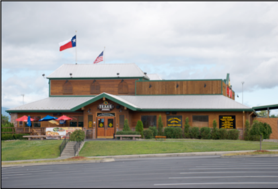
Do This: The Texas Roadhouse at Dena Marie Plaza utilizes natural materials such as cedar siding and brick and these materials are used for all exterior building walls and ancillary structures. The use of a metal roof on this building is appropriate given the building architecture. An earth tone green is utilized for the trim and building foundation plantings add visual appeal.
