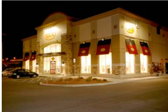
Do This: Night view of same building, which used to house the Talbot's Department Store. The architecture of the building incorporates horizontal and vertical variation and large windows to appeal and engage customer interest – especially at night. Well-designed buildings lend themselves to adaptive reuse
