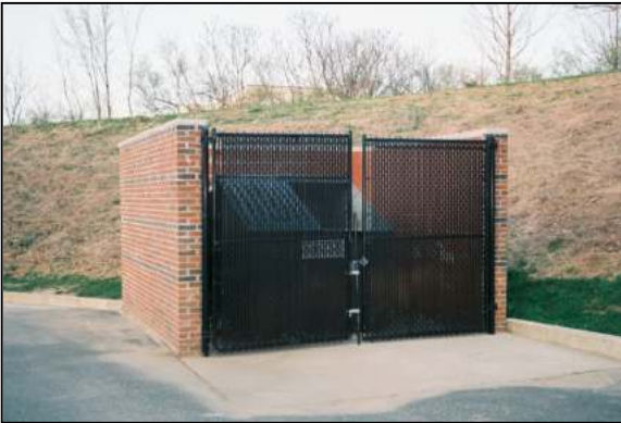
Do This: This dumpster enclosure is set on a concrete pad and enclosed on three sides with a brick wall. The doors for the dumpster enclosure utilize an opaque mesh to effectively screen the trash container, which is housed inside. This dumpster is also placed behind the commercial establishment where it is not visible from the public right-of-way.
