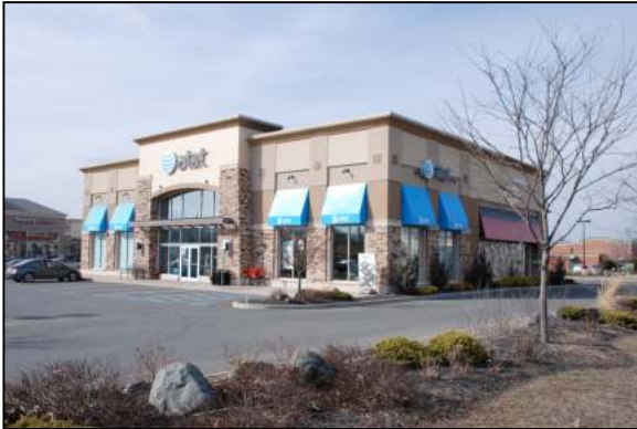
Do This: An AT&T Store in the Ulster Crossing Mall. The architecture of the building incorporates horizontal and vertical variation and a variety of durable building materials to create visual interest. The lower portion of the façade incorporates a faux stone façade, which is attractive and durable. The upper cornice accentuates the horizontal variation and adds visual interest.
