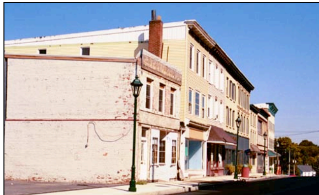
Above: Notice the pitched rooflines in each of these buildings which are concealed behind a parapet wall that also incorporates a decorative upper cornice.
