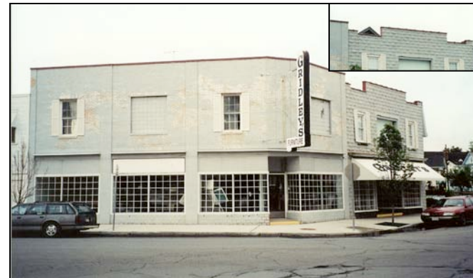
Above: The Gridley Building uses a parapet wall to conceal a pitched roofline [see inset].
