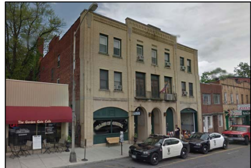
Above: Village of Catskill, Village Hall and Police Department. This historic building is home to Village government and is an important civic anchor on Main Street.
