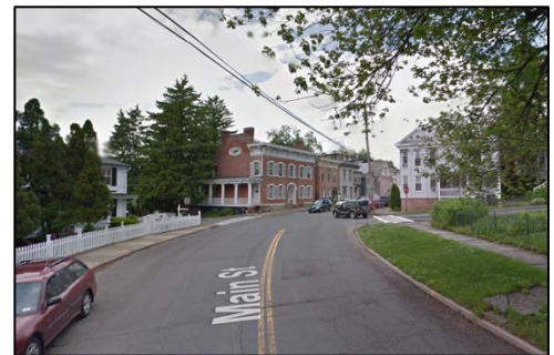
Above (top to bottom): View of sidewalk transition from standard 5-foot with to pathway just north of Marina Drive; view of substandard sidewalks between Marina Drive and Henry Street and view of transition back to standard sidewalks in the vicinity of Greene Street. There is a substantial need to improvements to sidewalk system between the waterfront and Downtown.
