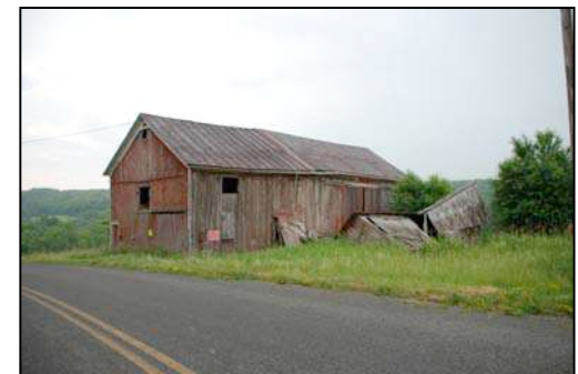
Above (top to bottom): Cold Spring Stock Farm (Lena Road) is an example of farm that is now owned by a second-homeowner; view of abandoned farmland at the Turnbull Road-Quinlog Road Wye; and view of abandoned barn and farmland on County Route 16 between Jones and Card Road. As these lands revert to second growth forest many scenic vistas within the Town will be lost.
