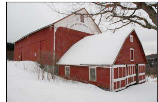
Above (top to bottom): Historic barn on CR 12 in the hamlet of New Lisbon; barn on Jones Road on property surrounded by Texas Schoolhouse State Forest; and barn at Cold Spring Stock Farm on Texas Road. Each of these barns helps to define the rich agricultural history of the Town and efforts to preserve these structures are strongly supported by this Plan.
