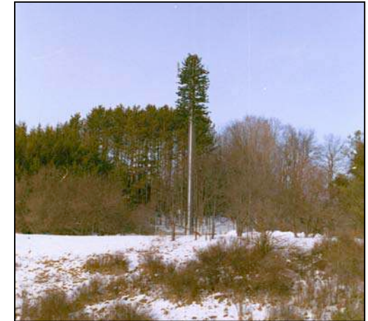
Photos (top to bottom): The Marcy-South power line has had a negative visual impact on the community - this Plan opposes situating like facilities in the Town; cellular communication tower in the hamlet of Livingston Manor, NY that is disguised as a pine tree. The cell tower design works since there are pine trees on this site. Cell towers have also been situated on silos.
