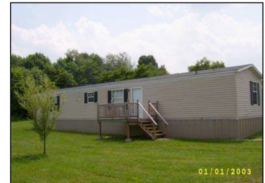
Above (top to bottom): Poorly placed and abandoned mobile home on CR 12 that has become an eyesore that adversely affects neighboring properties; poorly maintained mobile home and unregistered vehicles in the Town of Ulster, NY; and example of nicely situated mobile home in a rural community.
