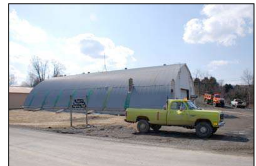
Above: Town of New Lisbon Highway Barn on CR 16 just to the south of the hamlet of Garrattsville. The useful life of this facility should be assessed in a Capital Improvement Plan (CIP).
