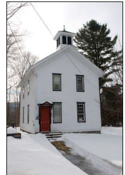
Above: The historic New Lisbon School District #2 Schoolhouse, circa early 1900’s on State Highway 51. The building is an excellent example of the vernacular architecture within the hamlet of Garrattsville.
