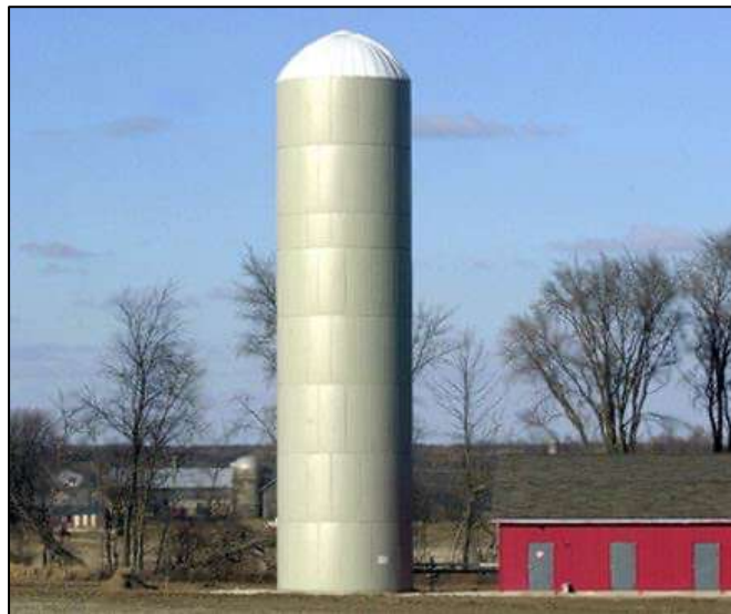
Above (left to right): Stealth Pine Tree cell tower and stealth silo cell tower and utility shed.
