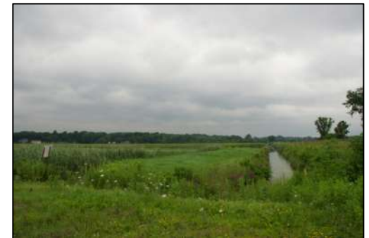
Above (top to bottom): Temporary pumping system for canal, which was utilized when pump stations were down (main pumps were down for two years between 2011 and 2013); view of outflow canal as it crosses under Lehigh & Hudson Rail Line and enters Camp LaGuardia; view of canal along Black Dirt field north of the Lehigh & Hudson Rail Line.
