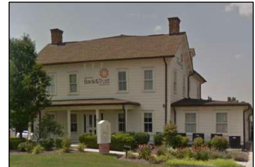
Above (top to bottom): The Tractor Supply Co. in the Chester Mall Shopping Center, Brookside Avenue (Route 17M); Outdoors, which is an outdoor sport shop situated at 6 Howland Street in Downtown; and Orange Bank & Trust Company on NYS Route 17M opposite the entrance to the Chester Mall.
