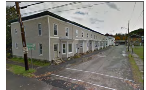
Above (top to bottom): View of well-maintained sidewalk segment in front of the State Theatre in the heart of the Downtown business district along Front Street; view of well-maintained ADA compliant sidewalks along both sides Court Street [between Front Street and Second Street] and view of poorly maintained sidewalks and drains along Church Street [between Front Street and Second Street] that are a deterrent to pedestrian travel. This Plan support complete street enhancements along this segment of Church Street.
