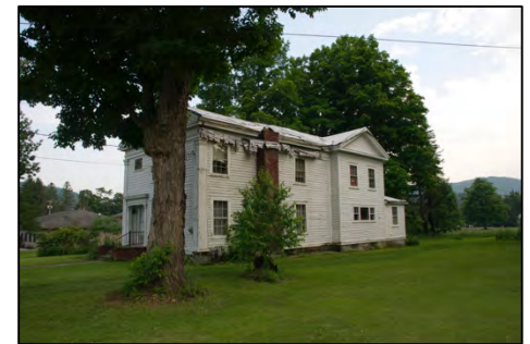
Above (top to bottom): A Classic Greek Revival home on Second Street in need of repainting and other repairs; another example of a Greek Revival home, this time showing a home that is in a serious state of disrepair with a leaking roof, loss of front porch overhand and neglected exterior. When historic properties are allowed to become dilapidated they diminish property values, while these same homes restored would dramatically increase property values in the Village.
