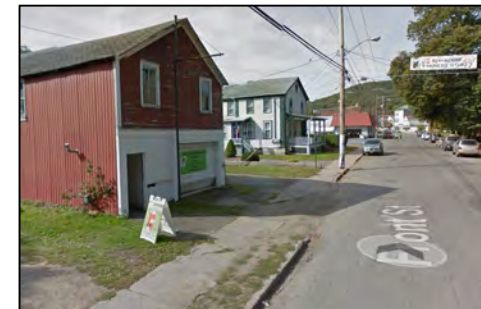
Above (top to bottom): Culvert crossing the Butler Brook at the corner of Division Street and Front Street that needs to be replaced (sidewalk is closed and weight limit posted); view of some segments of paving along Front Street that are beginning to crack and need to be sealed, and view of curbing, sidewalk and drainage deficiencies near the Front Street-Elm Street intersection. This Plan supports Village grant applications to secure funding to address these deficiencies.
