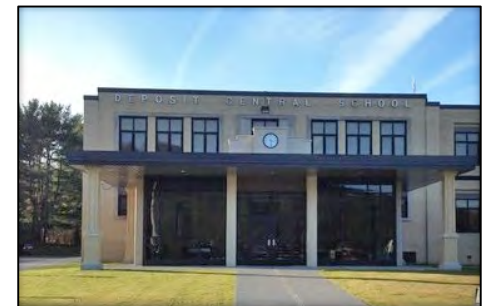
Above (top to bottom): Various images of the Deposit Central School buildings, which are situated within the Village of Deposit. The Deposit Elementary School, Middle School and High School are situated on a central campus on Second Street. The school contains a variety of athletic fields along with a community swimming pool that is managed by the Village along with the Towns of Deposit and Sanford. The Village has an excellent school system, but better employment opportunities are needed for graduates.
