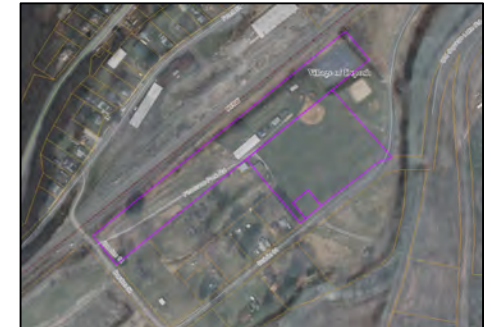
Above (top to bottom): Aerial view of Deposit Senior-Middle High School, which includes athletic fields and a community swimming pool that is operated during the summer with the cooperation of the Village of Deposit; aerial views of ball fields, basketball courts and volleyball court at Fireman’s Field Park, which is located on Dublin Street.
