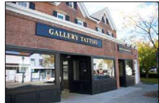
Above (top to bottom): View of Downtown mixed use buildings on Main Street; view of recently renovated Millspaugh Furniture store on Main Street with new upper cornice and large display windows; and view of renovation in progress for a new business to be called “Sweet Sensations By Sue”. Each of these appears to be eligible to be listed on the State or National Register of Historic Places. These photos illustrate renovations, which respect the original architecture of each building.
