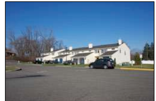
Above (Top to Bottom): Recently developed single-family home at the corner of Galloway Lane and South Montgomery Street, which is in the southwest quadrant of the Village; newer single-family residence off of Gate House Place in the northwest quadrant of the Village; and view of Winding Brook condominium development, which is also situated in the northwest quadrant of the Village of Walden.
