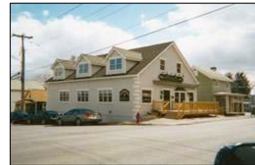
Above (top to bottom): View of one of the Jacobowitz and Gubits, LLP Law Office buildings on NYS Route 208 with its award-winning contemporary design; Thruway Shopping Center Plaza at base of Oak Street, Sweeney’s Tavern on NYS Route 208. Walden has a wide variety of business establishments that serve local residents and the surrounding region.
