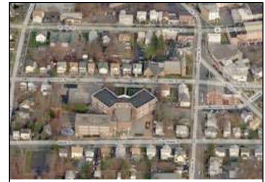
Above (top to bottom): Village’s WWTP on Bradley Lane, DPW Garage on Bradley Lane and view of street system near Elementary School. “Complete Streets” designed and operated to enable safe, attractive, and comfortable access and travel for all users including pedestrians, bicyclist, motorists and public transport is supported by this Plan.
