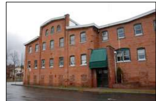
Above (top to bottom): View of Rider-Ericsson Company (aka Package Lighting Building) circa late 1800’s, looking south from Grant Street; view of workers housing along Railroad Avenue and view of Wooster Manufacturing Company (aka Nelco Building) circa 1876. Each of these buildings appears to be eligible for listing on the State or National Register of historic buildings and perhaps district designation.
