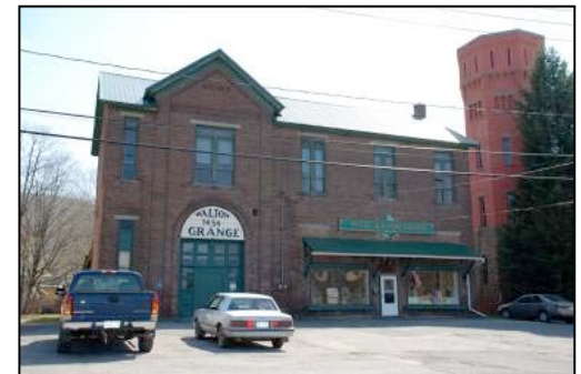
Above (top to bottom): Hess Gas Station on Delaware Street; Offices of the Delaware County Soil & Water Conservation District; the Walton Grange Building that lies to the south of the West Branch of the Delaware River on Stockton Avenue. The Water Street Wells are located in an urbanized area with many potential contaminant sources and large expanses of impervious surfaces.
