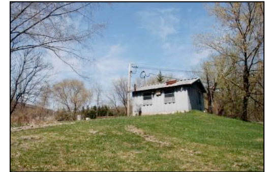
Above (top to bottom): View of the County Department of Public Works storage yard as seen from the edge of the Water Street Well Building berm; view of access driveway into the Water Street Well Field; view of Water Street Well Field Well Building looking south toward the West Branch of the Delaware River showing the raised berm to get above the floodplain.
