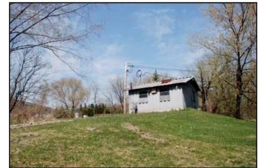
Above (top to bottom): The Village Water Storage Tanks that are situated on a ridge above the Village so that they also provide sufficient pressure for fire suppression; view of Austin Lincoln Park Well Head near baseball field; view of Water Street Well Field Well Building. Notice that the well building is situated on a raised bed to bring it above the floodplain.
